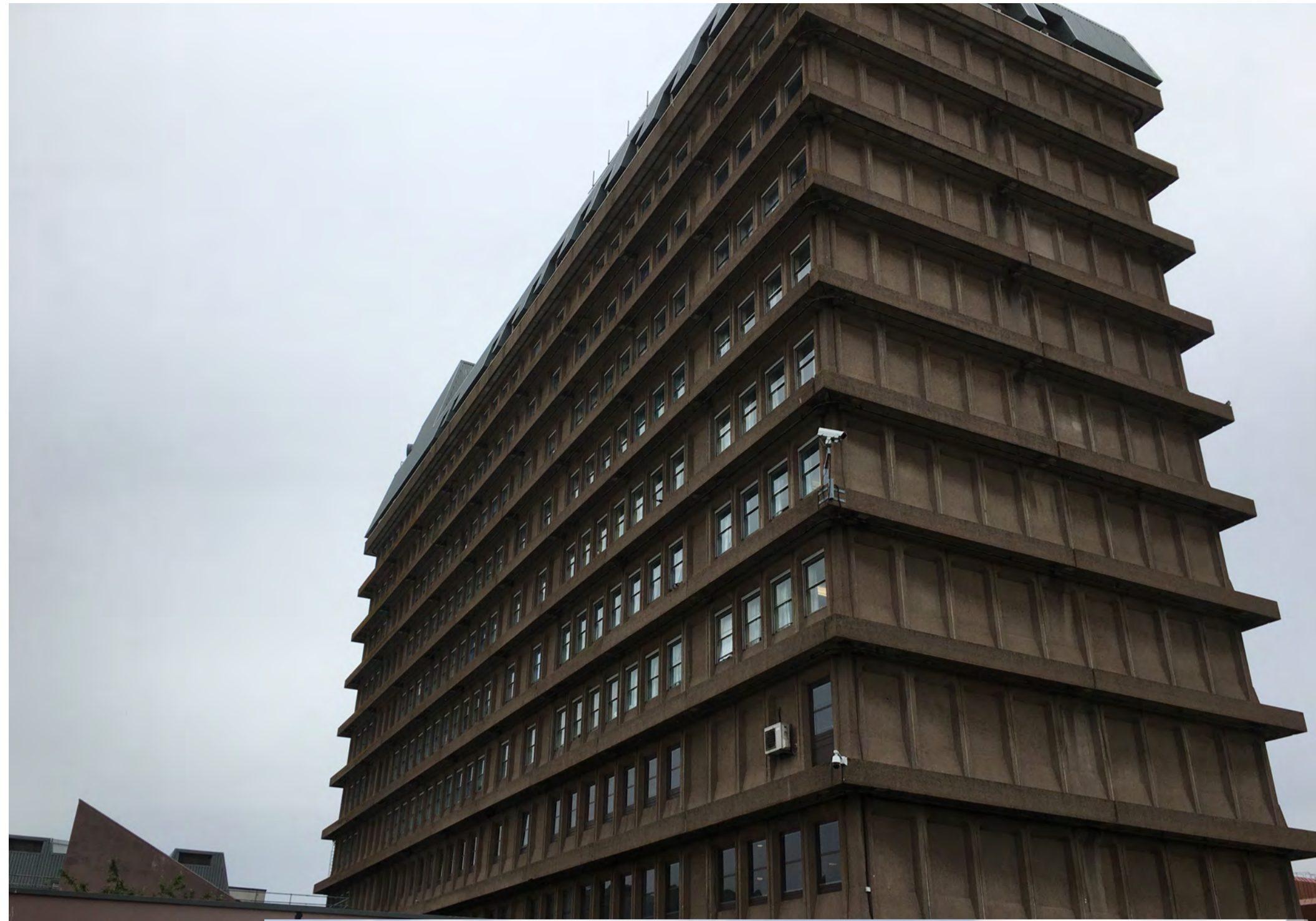
EXISTING VIEW FROM SOUTH WEST
