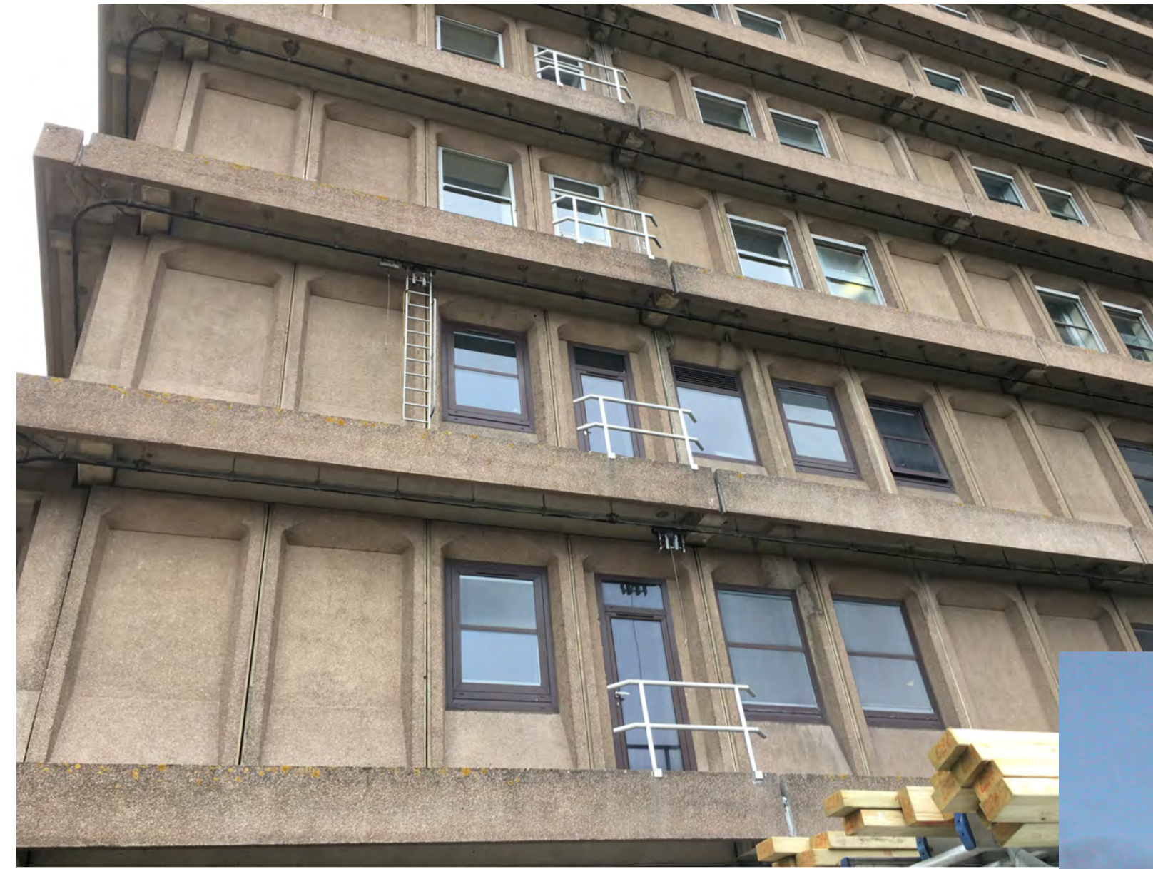
EXISTING DETAIL VIEW
